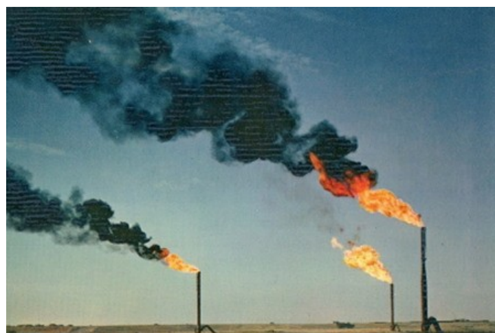
Torchères, photo SN REPAL
